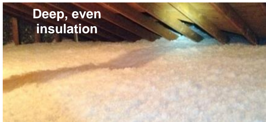
Figure 8. High-quality blown-in attic insulation
